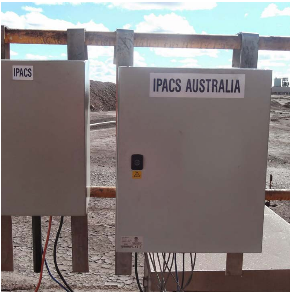
Figure 4. Installation of IPACS condition monitoring on site. (Clockwise from top left) a. sensor install b. camera install c. overview of the conveyor drive with main stockpile in background d. networking (left) and sensor processing cabinets (right)
