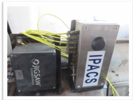
Installation of the IPACS remote monitoring box inside the driver cabin
